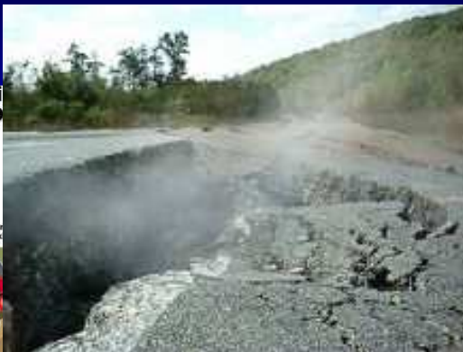
Pillars of coal collapse, damaging streets and structures
